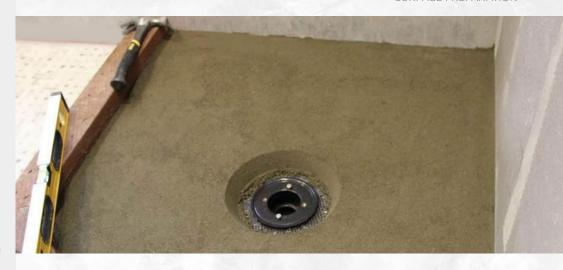
Siena Deck Mud is a factory blended mortar bed consisting of portland cement which complies with ASTM C150 and graded sand which complies with ASTM C144. Siena Deck Mud is designed to create a high strength mortar bed for horizontal applications of most tile or stone installs. Siena Deck Mud can also be used to create a new substrate, fill or raise an existing substrate.
