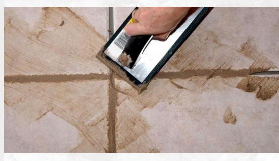
Siena Sanded Grout GS300 is a polymer-enhanced premium grout manufactured with a mixture of portland cement, very fine graded aggregates and other proprietary additives to produce a high quality grout that requires only the addition of water. Siena Sanded Grout GS300 is mildew resistant, efflorescence resistant, available in 36 premium colors, and complies with the requirements of ANSI A118.6.
